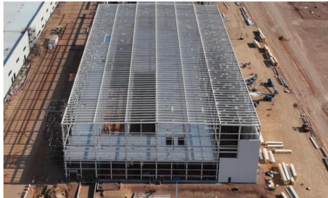
Paint: Steel erection and wall siding installation
