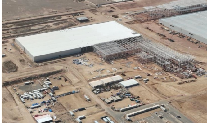
Body-In-White: Wall siding, roof metal decking Installation
